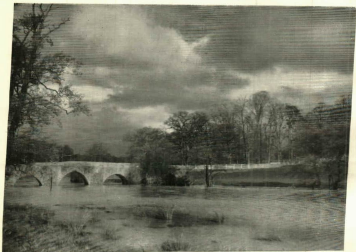
TESTON, NEAR MAIDSTONE XVth century bridge over River Medway
